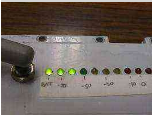
Power on. The first green LED is a battery indicator, the next two are lit because of background RF noise.
